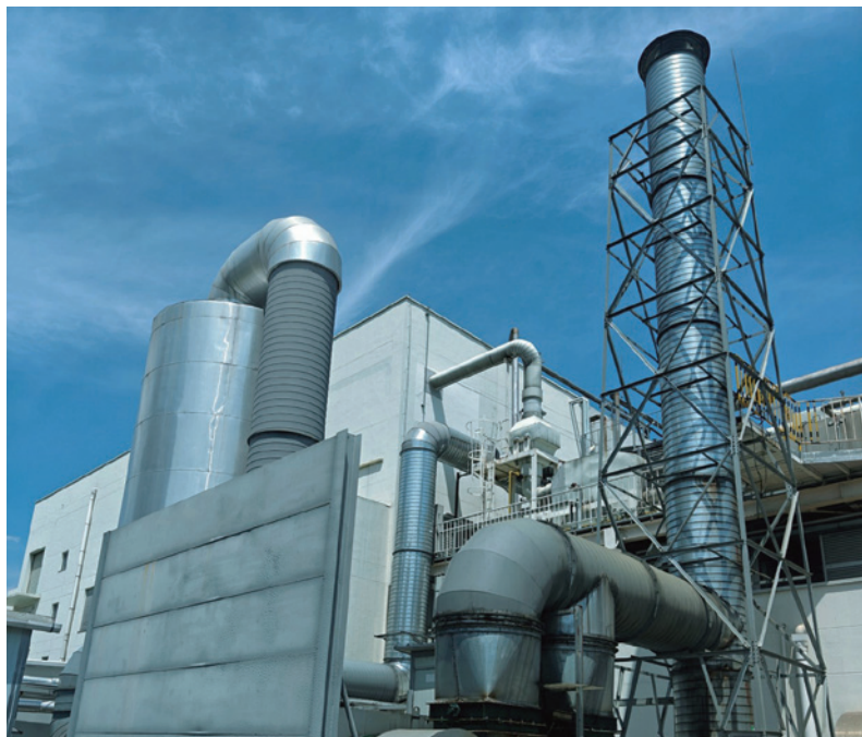
Exhaust gas treatment system (China Plant)
